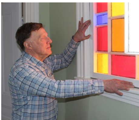
Dan Shagoury checks the fit of one of his new window inserts.
