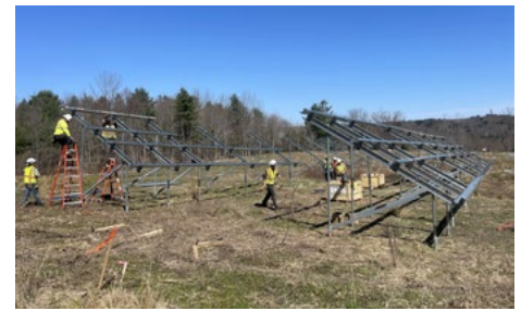
Perennial crew beginning installation of the Stevens Commons array.
